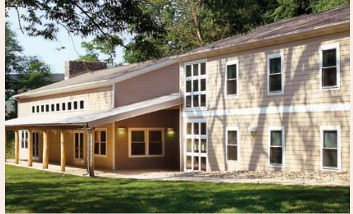
Photos Courtesy: Reward Wall System
